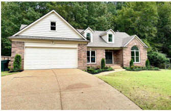
Front Of Structure
